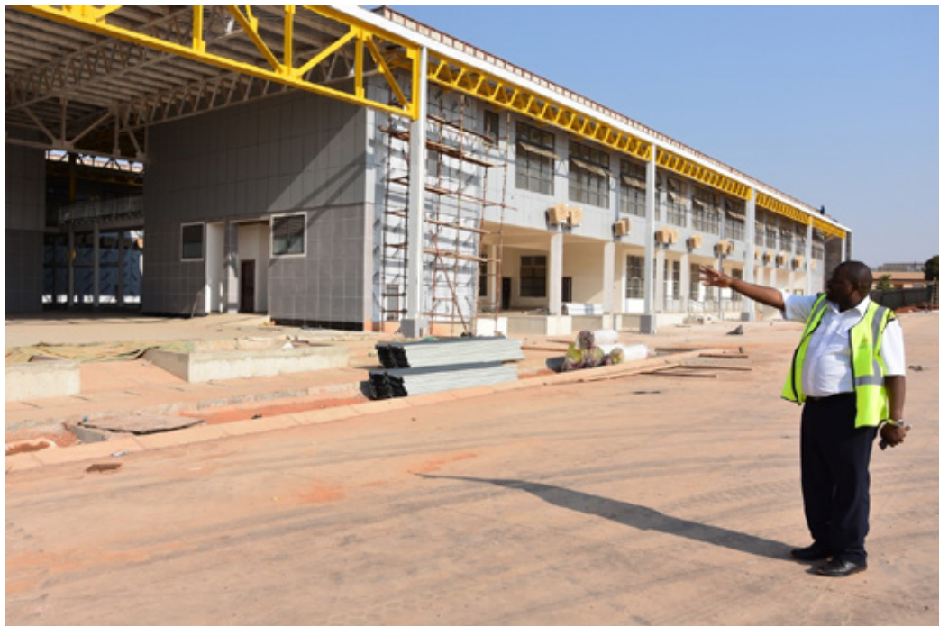
Mwami OSBP infrastructure under construction
