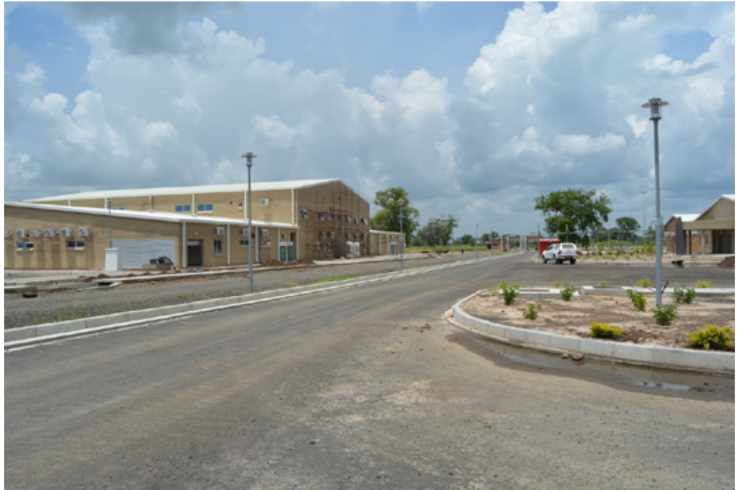
Part of Kazungula OSBP infrastructure
